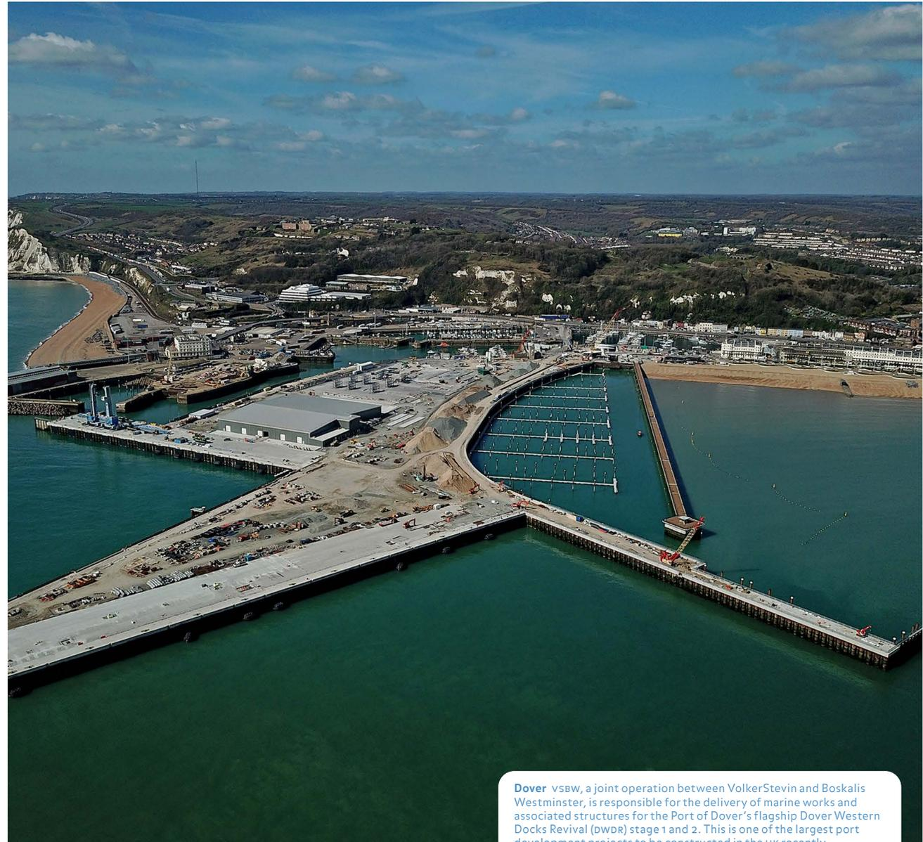
**Dover** vsw, a joint operation between VolkerStevin and Boskalis Westminster, is responsible for the delivery of marine works and associated structures for the Port of Dover's flagship Dover Western Docks Revival (DWR) stage 1 and 2. This is one of the largest port development projects to be constructed in the UK recently.
