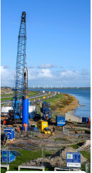
**Fryslân wind farm** Visser & Smit Hanab delivering Horizontal Directional Drilling of around 1370 metres for Windpark Fryslân.
