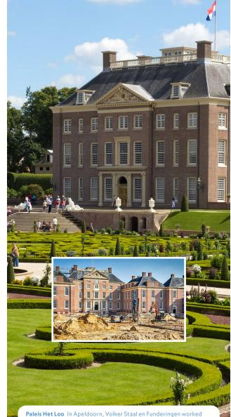
Paleis Het Loo In Apeldoorn, Volker Staal en Hunderingen worked for a year on the underground expansion of the Paleis Het Loo museum. A ten-metre deep excavation pit has been constructed, part of which runs underneath existing monument buildings. The palace, which is over 300 years old, has withstood the drastic underground work without sustaining any damage.
