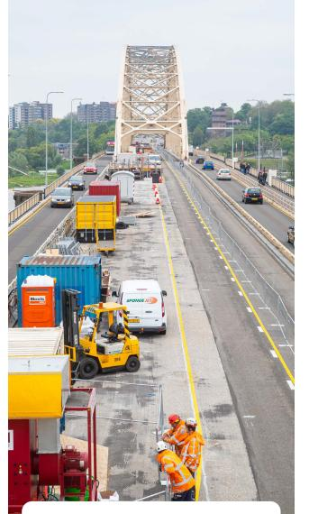
Waalbrug Renovation of the 80-year-old Waalbrug bridge at Nijmegen is necessary to ensure smooth and safe traffic across the bridge in the future. kws is responsible for the renovation of the concrete deck, the painting of the steel structure and the conversion of the bus lane into a cycle path. In the meantime, as much traffic as possible is allowed to pass through.
