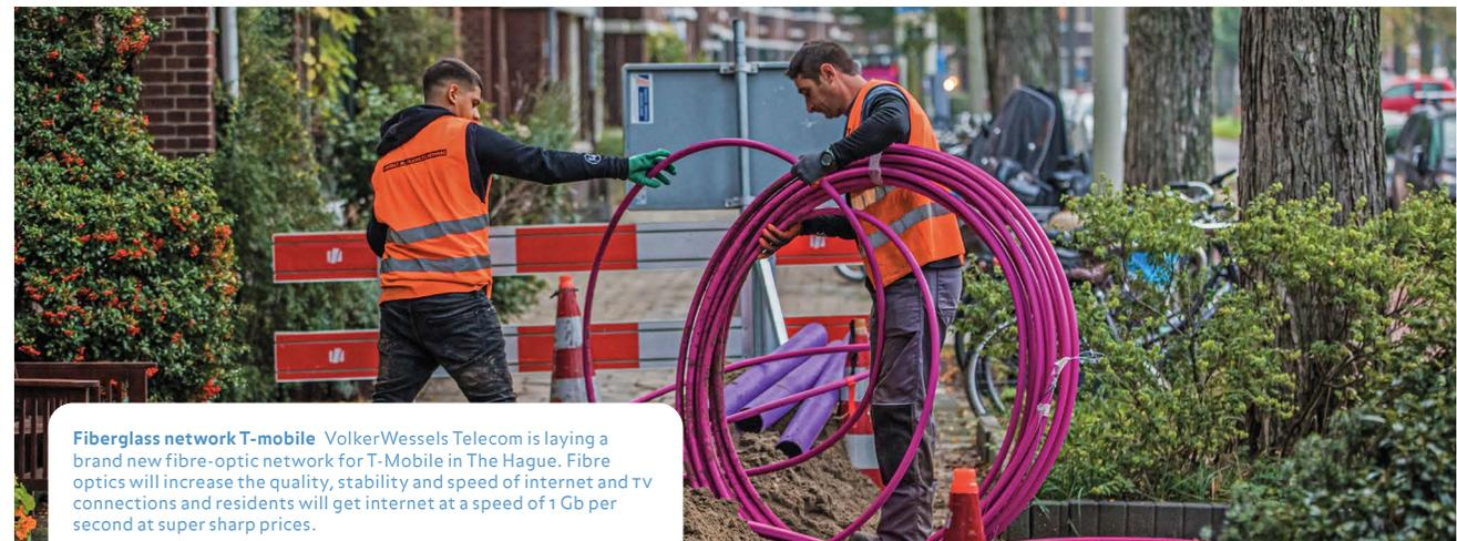
**Fiberglass network T-mobile** VolkerWessels Telecom is laying a brand new fibre-optic network for T-Mobile in The Hague. Fibre optics will increase the quality, stability and speed of internet and TV connections and residents will get internet at a speed of 1 Gb per second at super sharp prices.
