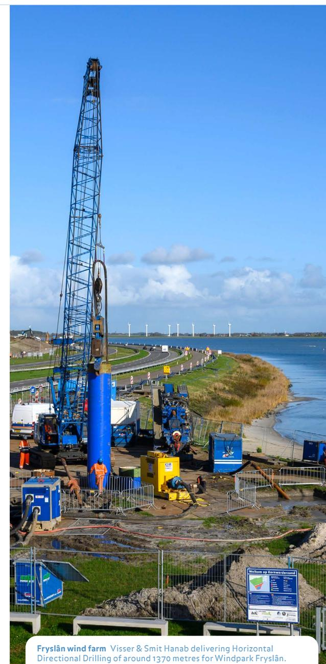
Fryslân wind farm Visser & Smit Hanab delivering Horizontal Directional Drilling of around 1370 metres for Windpark Fryslân.
