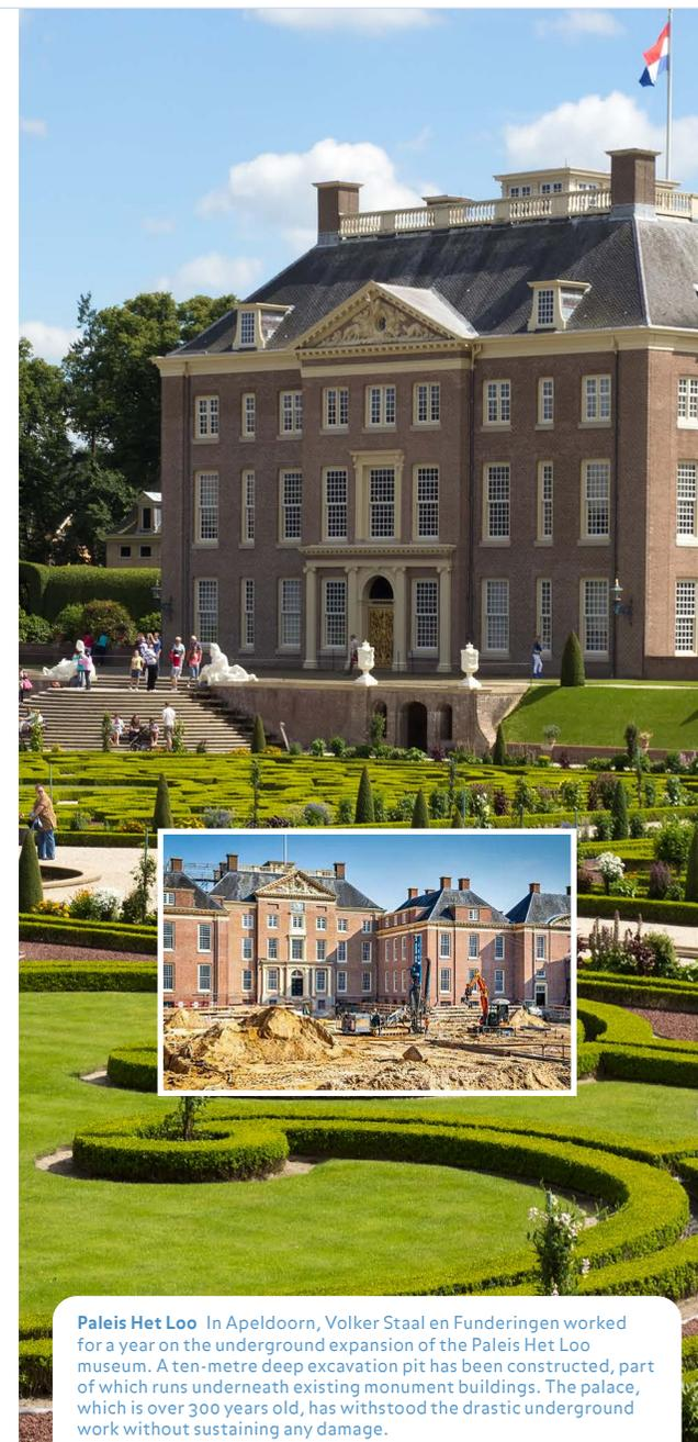
**Paleis Het Loo** In Apeldoorn, Volker Staal en Funderingen worked for a year on the underground expansion of the Paleis Het Loo museum. A ten-metre deep excavation pit has been constructed, part of which runs underneath existing monument buildings. The palace, which is over 300 years old, has withstood the drastic underground work without sustaining any damage.
