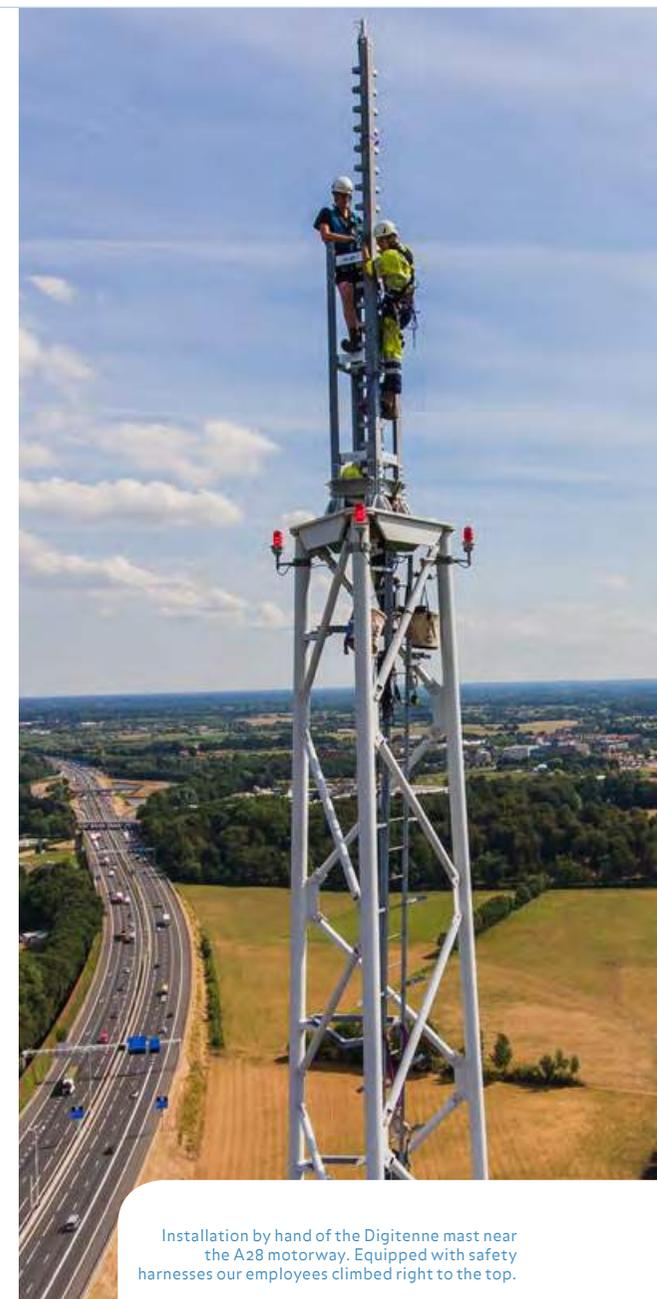
Installation by hand of the Digitenne mast near the A28 motorway. Equipped with safety harnesses our employees climbed right to the top.
