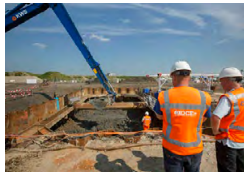
OCE, part of kws Infra, working at Badhoevebogen.
