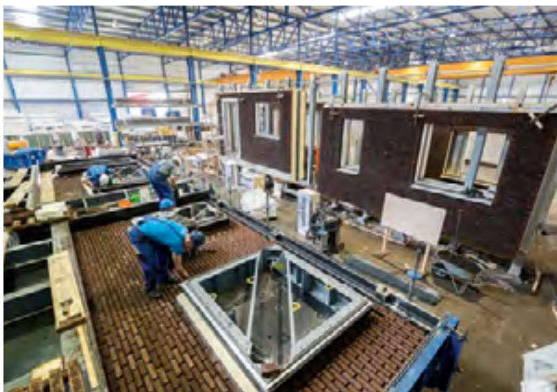
Prefabricated building elements for MorgenWonen (Future Living) were assembled at Westo.
