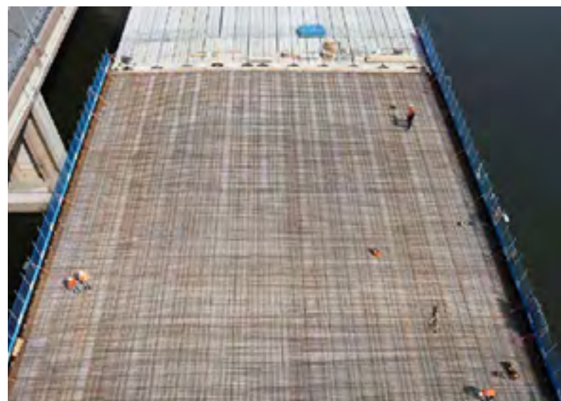
Working on a second Hollandse Brug bridge.
