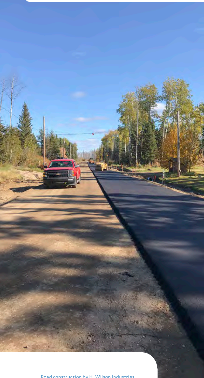
Road construction by H. Wilson Industries.
