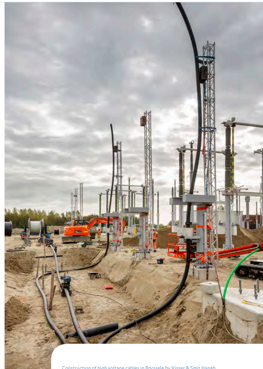
Construction of high voltage cables in Borssele by Visser & Smit Hanab.
