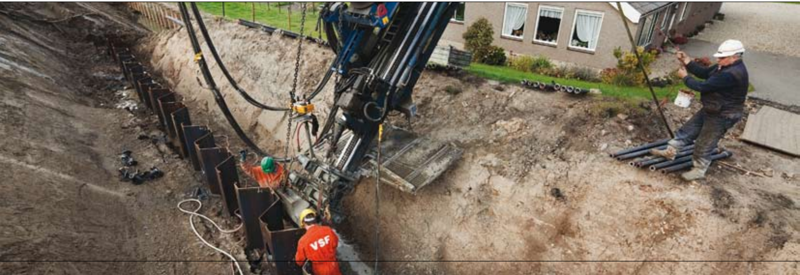
Anchored dam wall for dike improvement in Lekkerkerk
