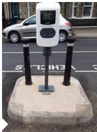
Installation of EVCP for Liberty Charge
